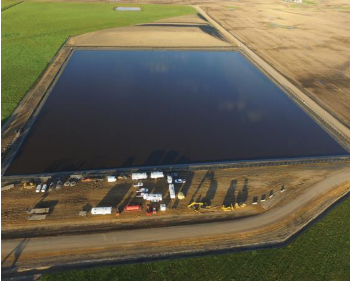
14-19-079-12W6 Water Storage Reservoir
